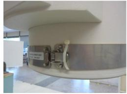
Philips urgently asks users of the affected device to fix the closed latch body of the draw latch to the metal band using a tie wrap. This will eliminate any immediate risk to the patient. Without such temporary measure, the device should not be used.
